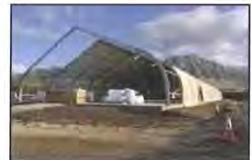
This temporary homeless shelter is taking shape in Wai'anae. Metcalf Construction is building the sprung structure ? it will be 70 feet wide, 270 feet long ? in a lot near Wai'anae Intermediate School.
